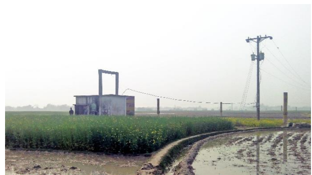
Photo.2 Grid connected pumping system
