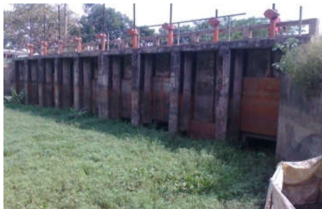
Figure 13 Sluice Gate at Amvita and Silted up Hamkura River (May, 2012)
