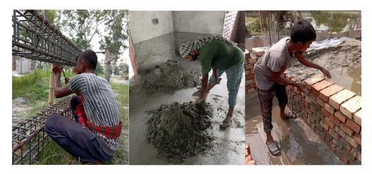
Figure 1: Workers doing Beam and column casting (Left side), Sand and cement mixing (Middle) and Masonry (Right side) work in awkward posture.
