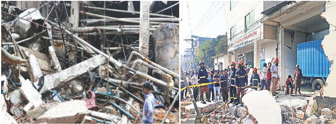
Figure 2: Boiler explosion at Multifabs Ltd on July 3, 2017 (Left) (“Boiler explosion”, 2017), and at Natural Sweater Village Ltd on December 10, 2019 (Right) (“One killed”, 2019)
