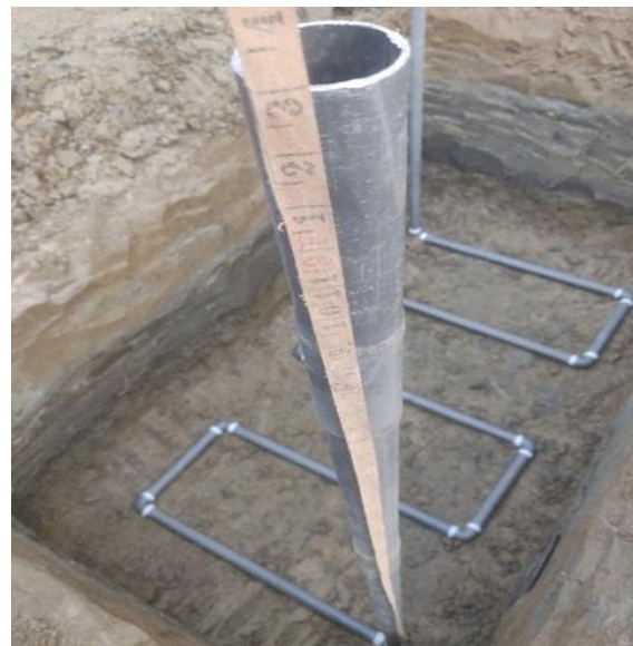
Figure 3: Pipe loop installation for EWPHE system
